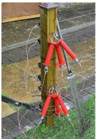
**5. It is now safe** to unclip the entrance wires and relocate on the hooks provided on the adjacent wooden posts.
